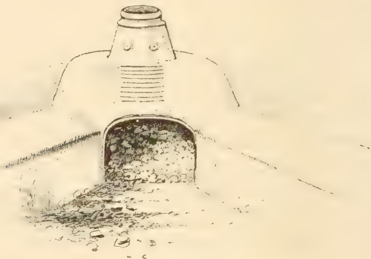
MAKALANGA IRON SMELTING FURNACE
